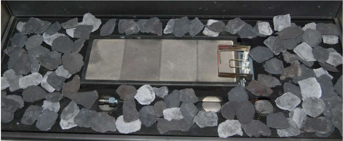
Photo 6 – Vermiculite chips spread around the burner
